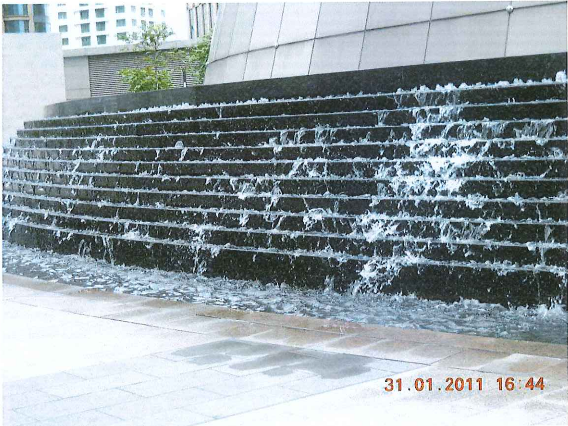
Picture 19: Water feature with granite finish including under water light
