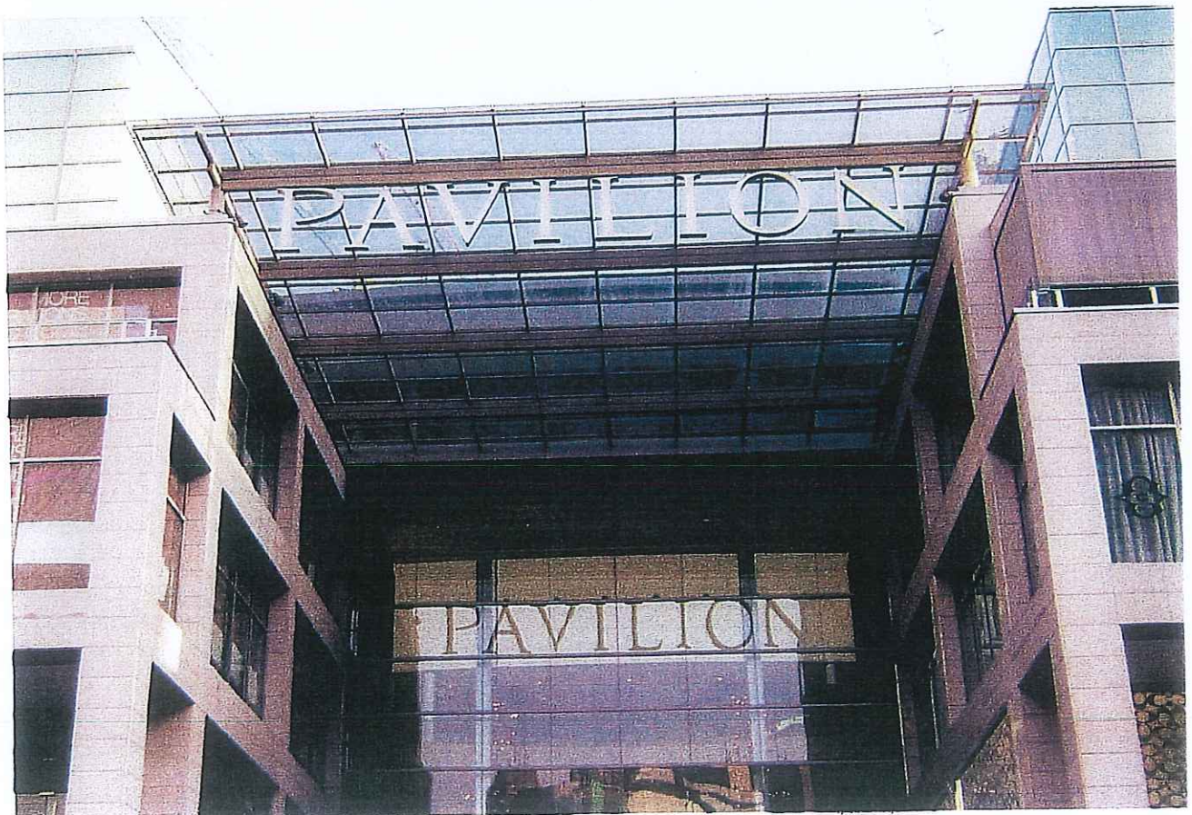
EXTERNAL FACADE CONSTRUCTION
