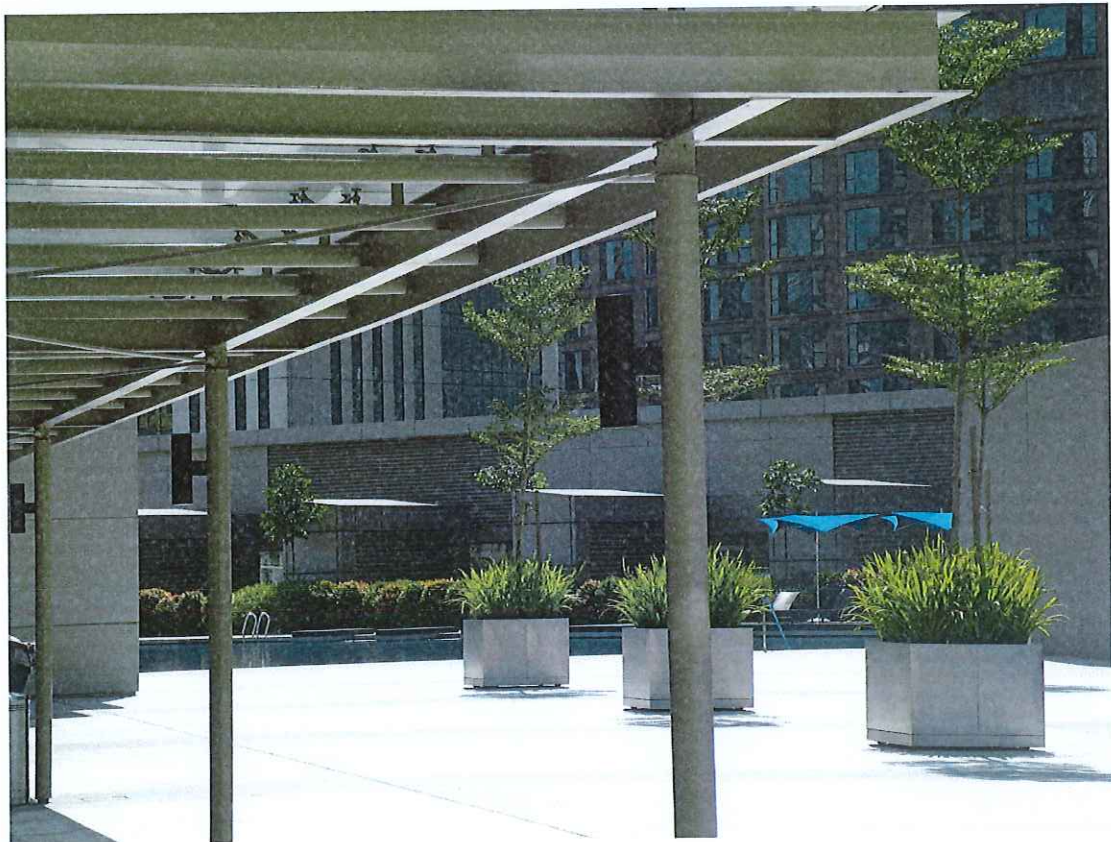
Picture 10: Stainless steel planter box & granite paving
