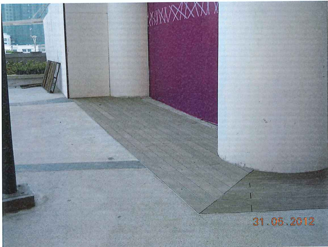
Picture 16: Composite decking & pebble wash floor finished
