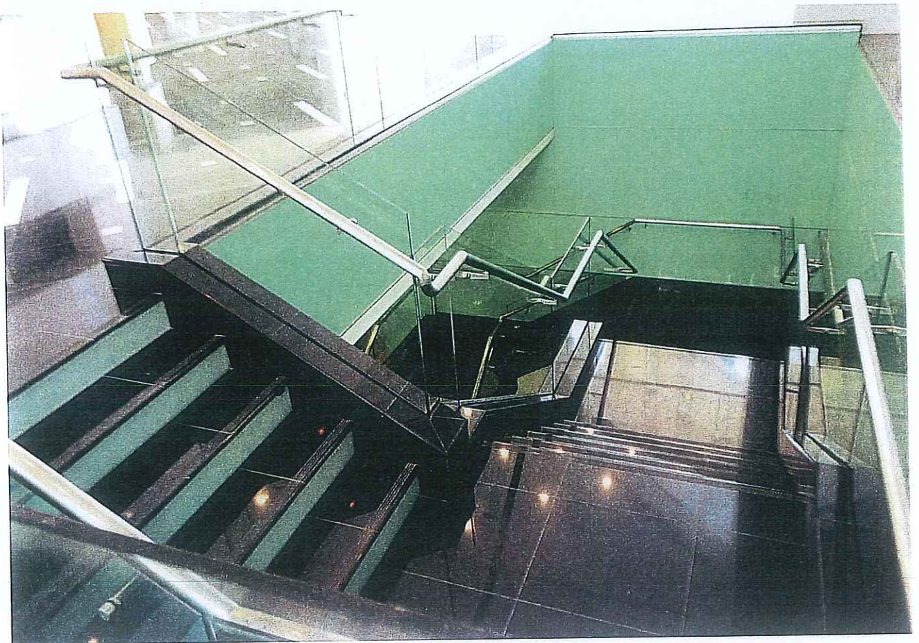
DIMENSION STONE TO STAIRCASE
