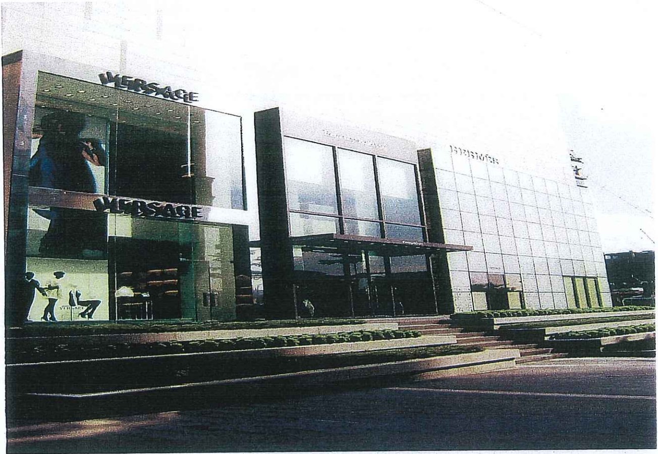
EXTERNAL FACADE CONSTRUCTION
