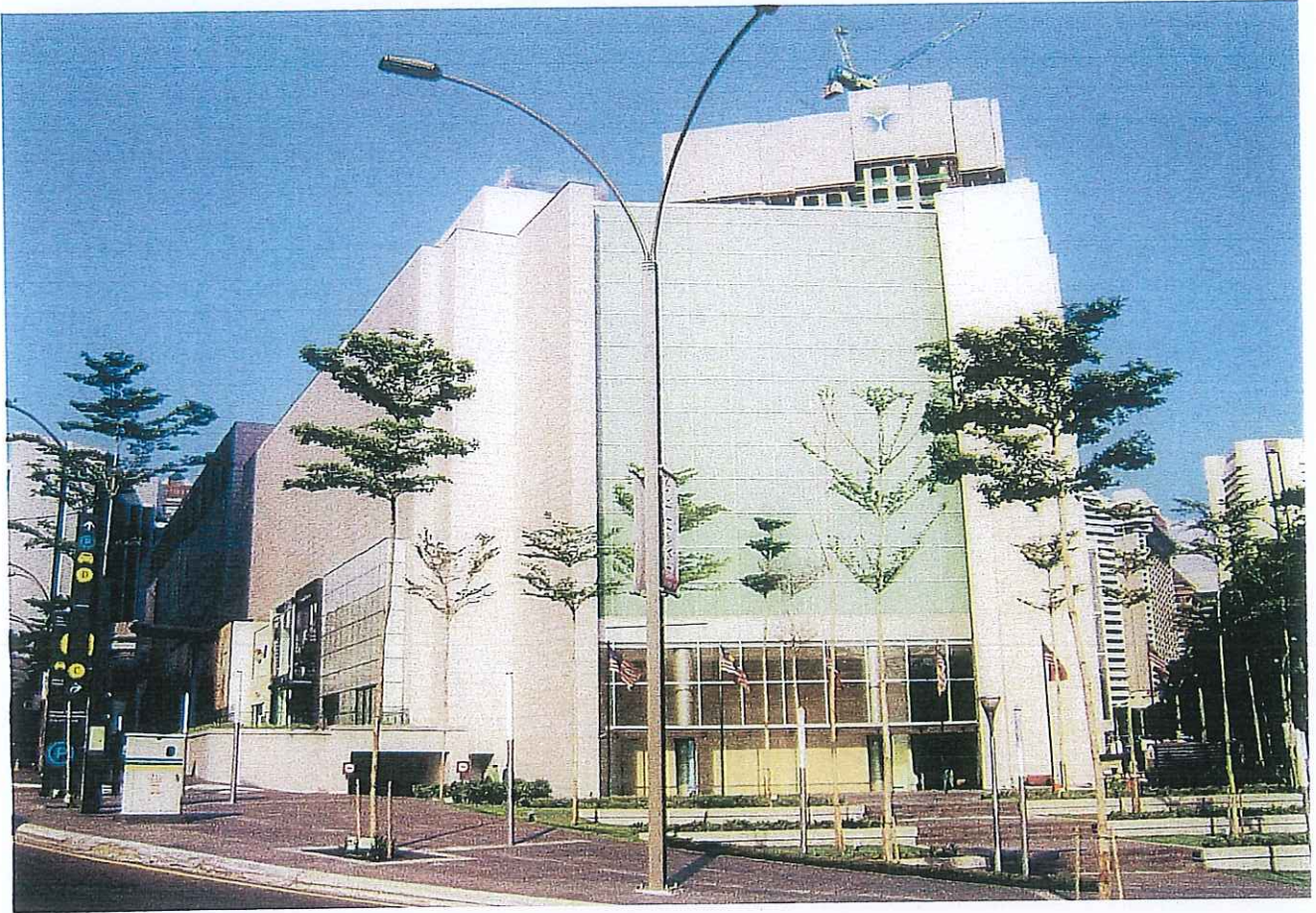
EXTERNAL FACADE CONSTRUCTION
