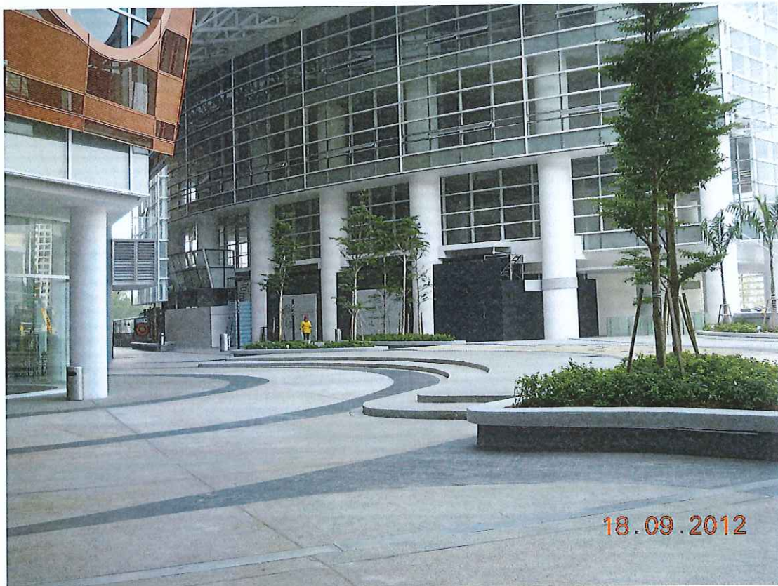
Picture 18: Pebble wash floor with granite insert pattern
