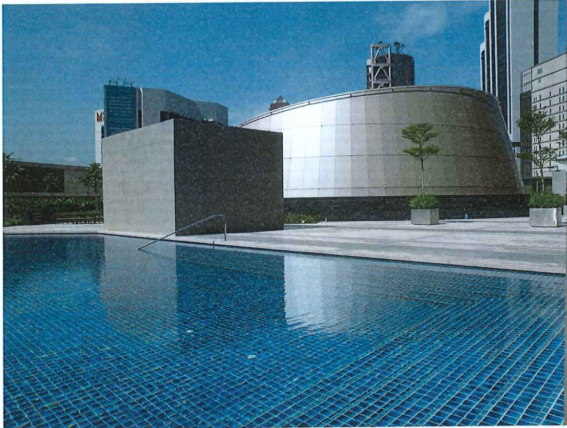
Picture 7: Thai mosaic tiles at swimming pool
