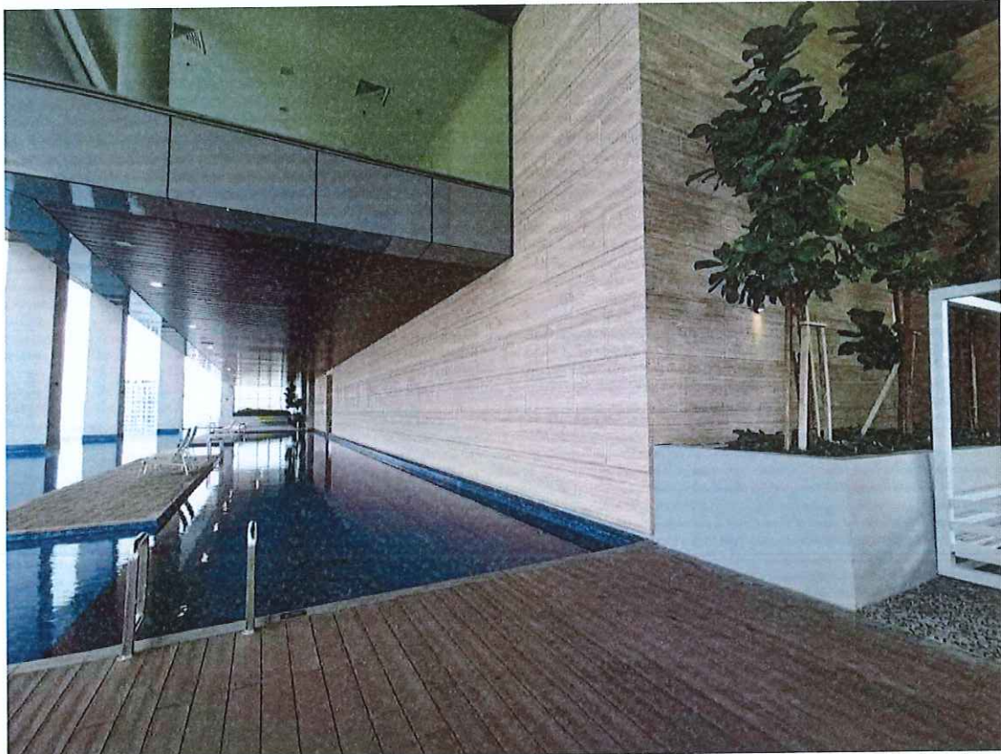
Picture 11: Travertine Wall Cladding and timber deck
