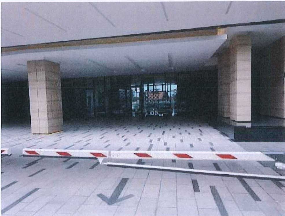
Picture 4: Travertine Column & Granite Paver at Drop Off Area
