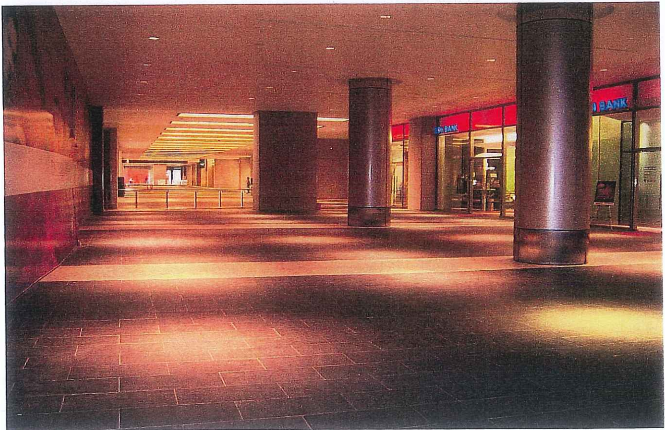
GRANITE FLOOR & WALL FINISHES
