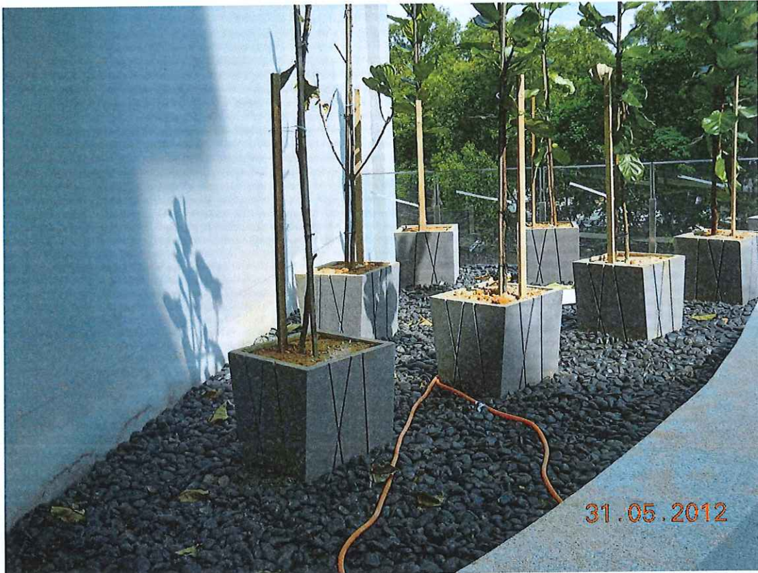
Picture 17: Loose river stone and GFRP planter box
