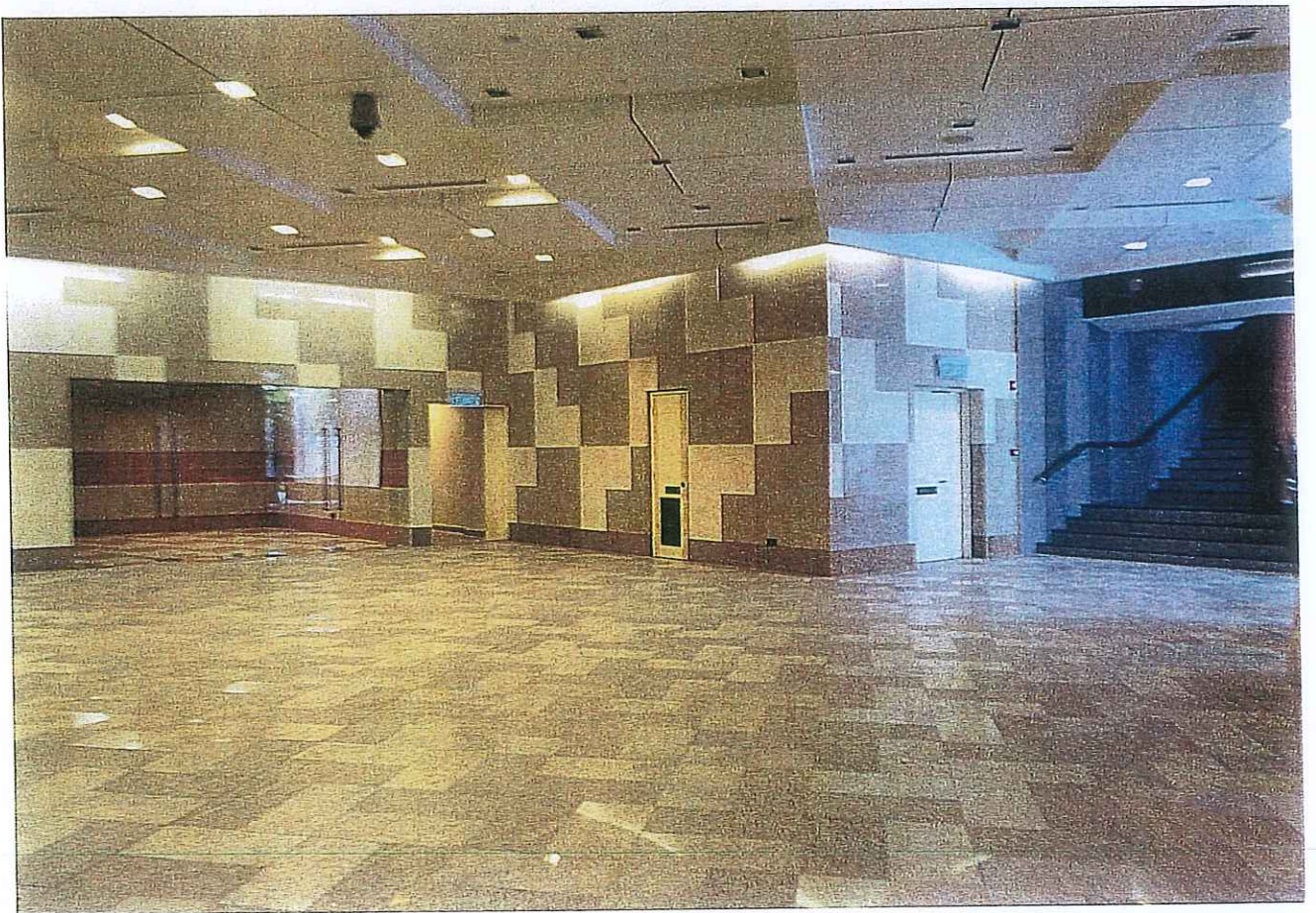
DIMENSION STONE TO MAIN LOBBY
