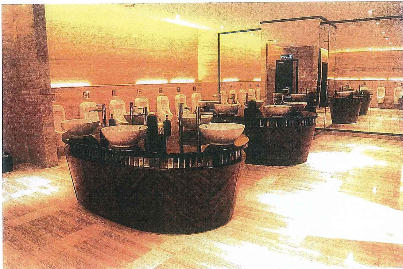
DIMENSION STONE AT WASH ROOM
