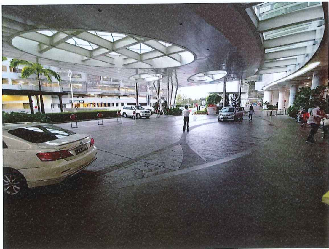
Picture 12: Concrete Imprint, pebble wash and granite paving
