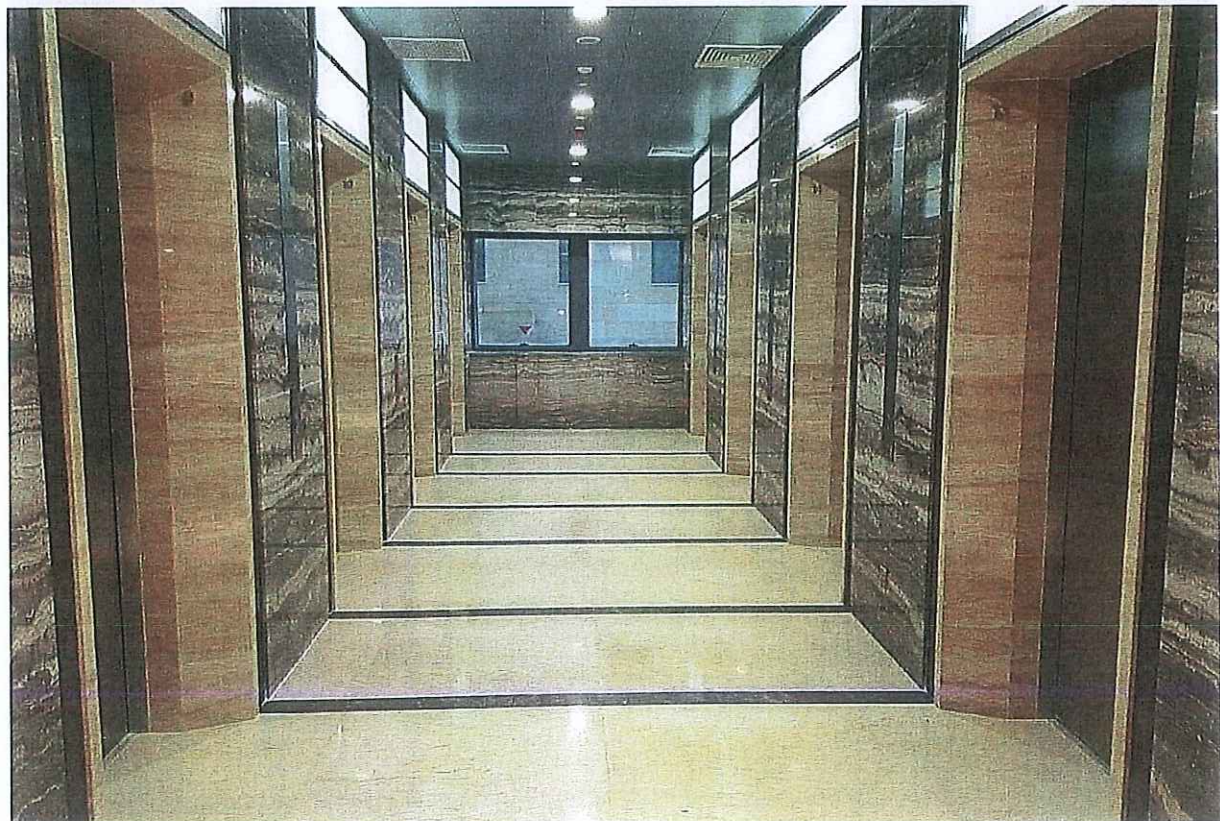
DIMENSION STONE AT LIFT LOBBY
