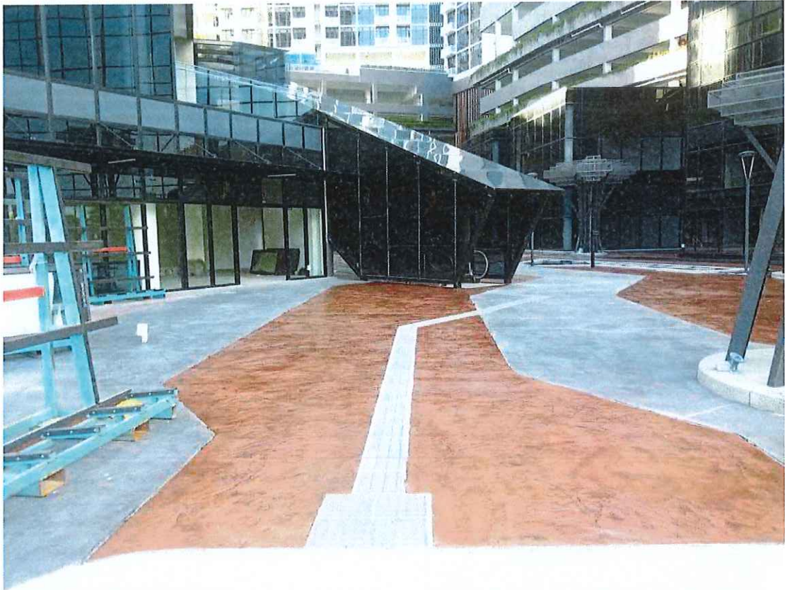
Picture 21: Concrete imprint
