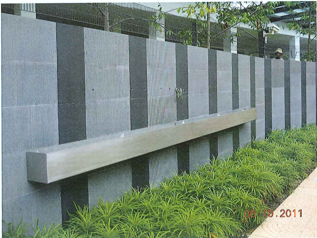
Picture 24: Stainless steel planter box & fencing wall
