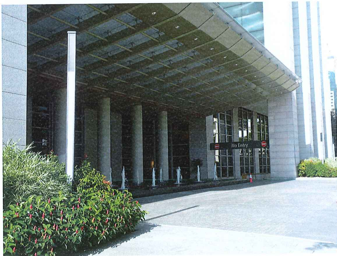
Picture 4: Water Feature, driveway granite
